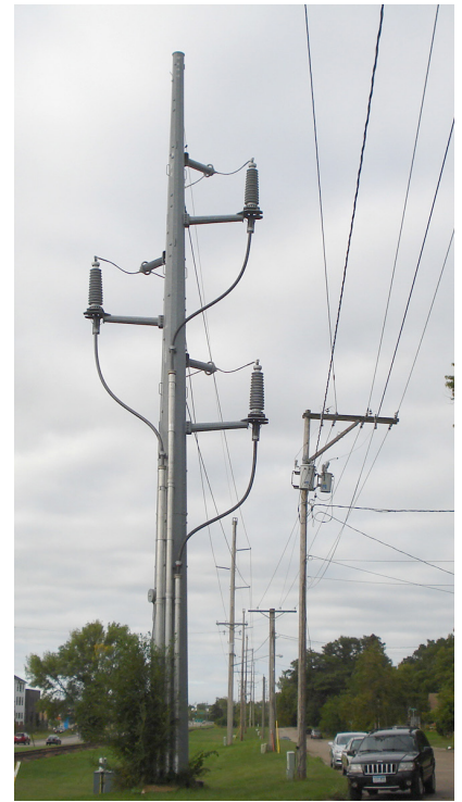
Example of a steel underground termination structure. Photo courtesy of POWER Engineers, Inc.
