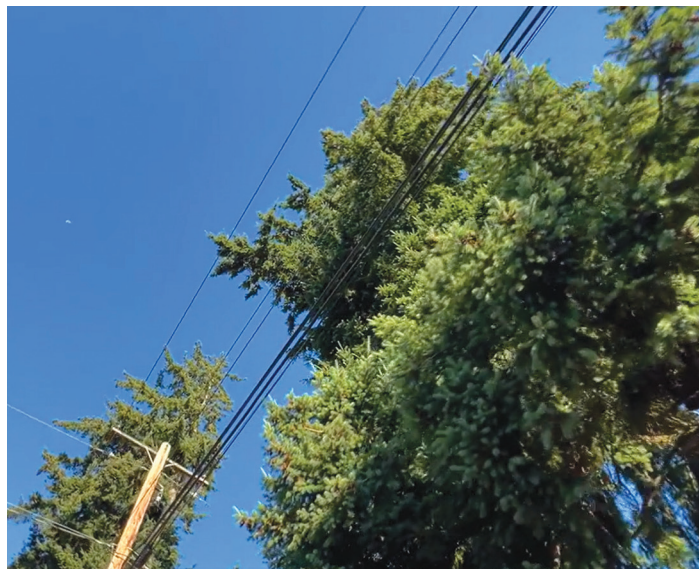
Example of trees that have grown into a power line and need to be trimmed.
