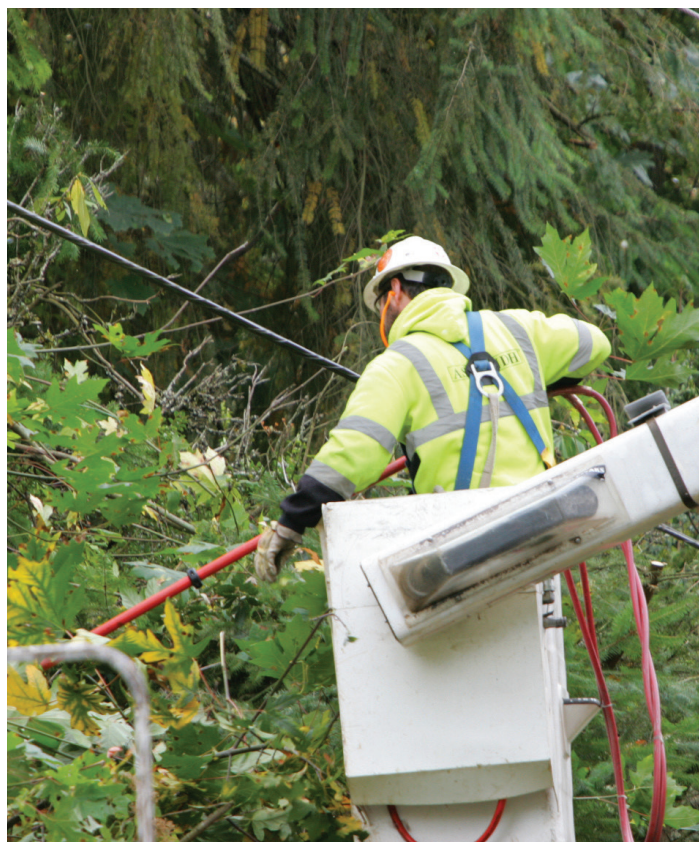
Trimming limbs that have grown too close to power lines.
