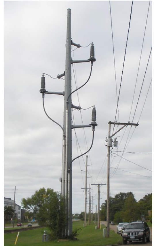
Example of a steel underground termination structure. Photo courtesy of POWER Engineers, Inc.
